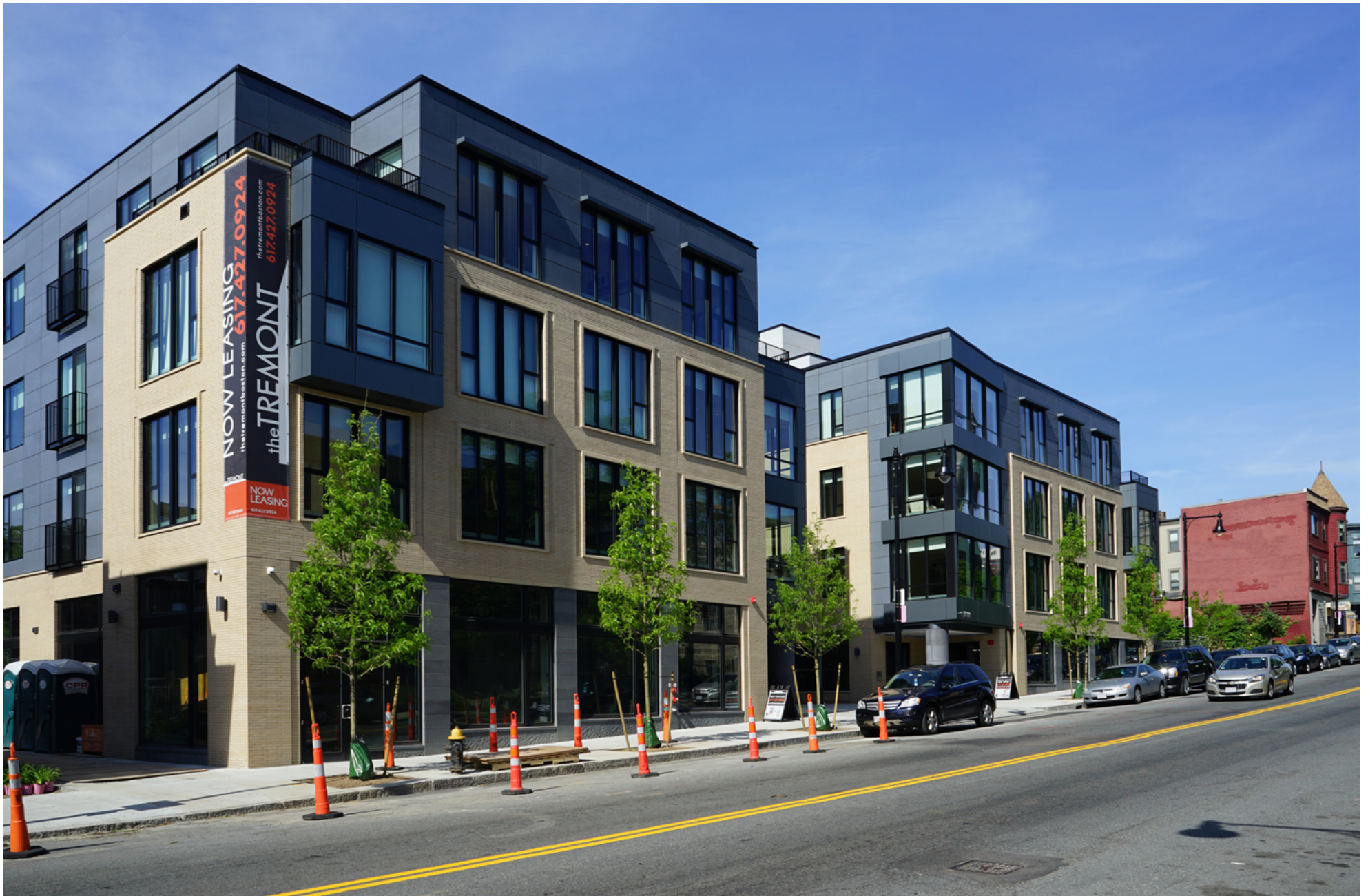
The Tremont looking southwest.
