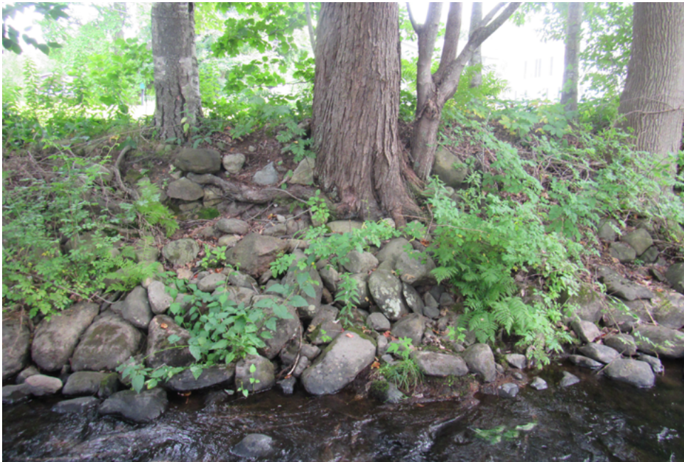
Stone bank protection on the right bank of the channel, across from the tannery site. Bank hardening, which is present on both sides of the channel, is a legacy of the river's industrial past that impairs habitat quality.
