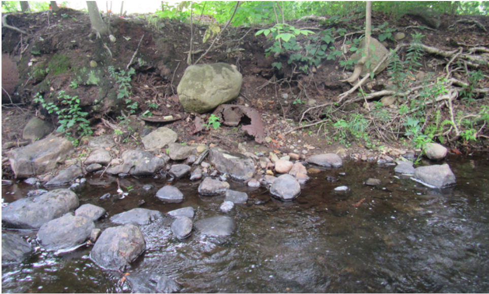
Remnants of a buried tank on the left bank of the channel. The tannery site is in the background.
