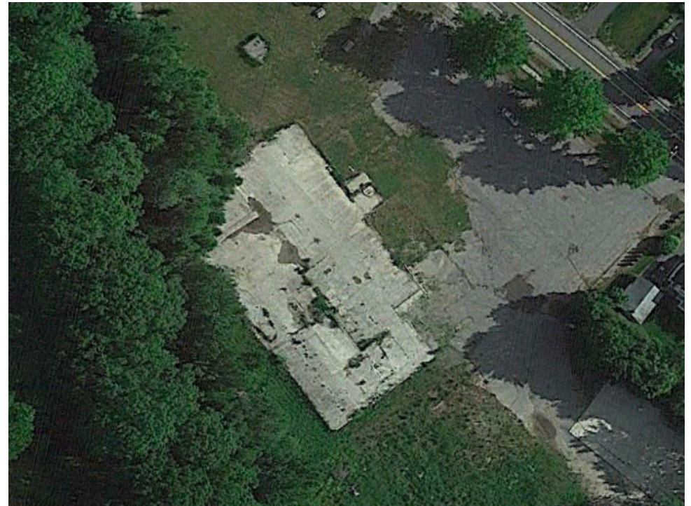
Existing concrete slab on the site leftover from the former Apollo Tannery.
