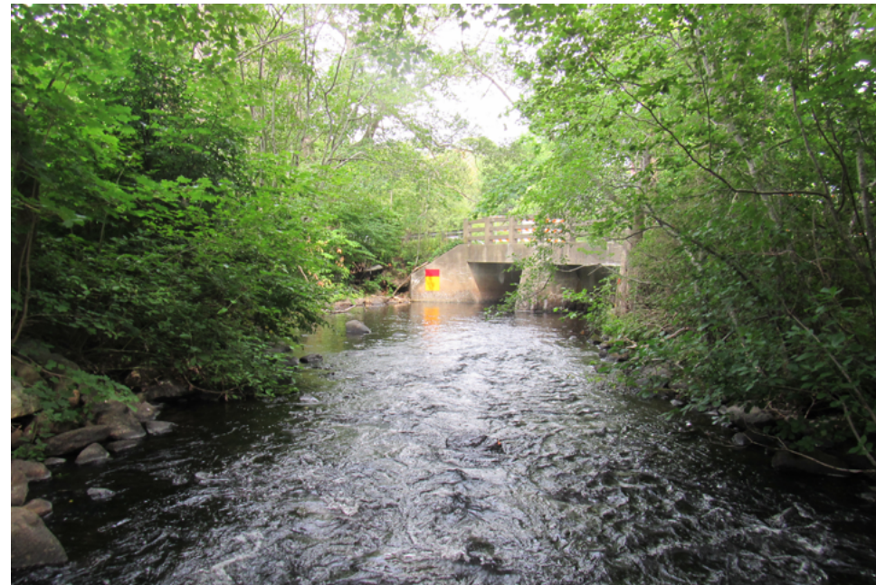
Looking downstream towards the lower end of the reach at the Rawson Avenue crossing. The tannery site is to the left of the photo.
